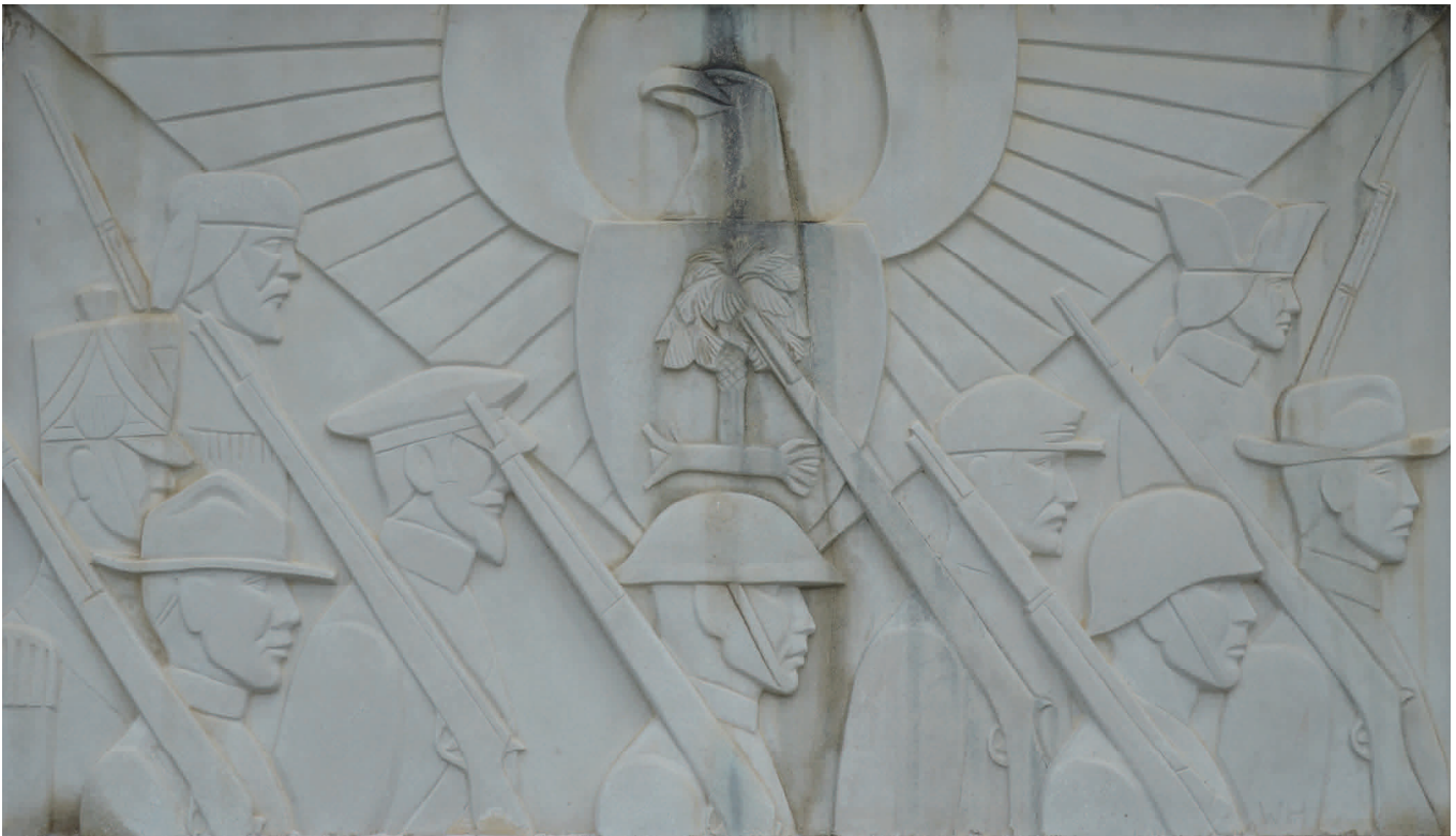
Figure 2. Hirsch panel at the Barnwell Armory as it appears today.
