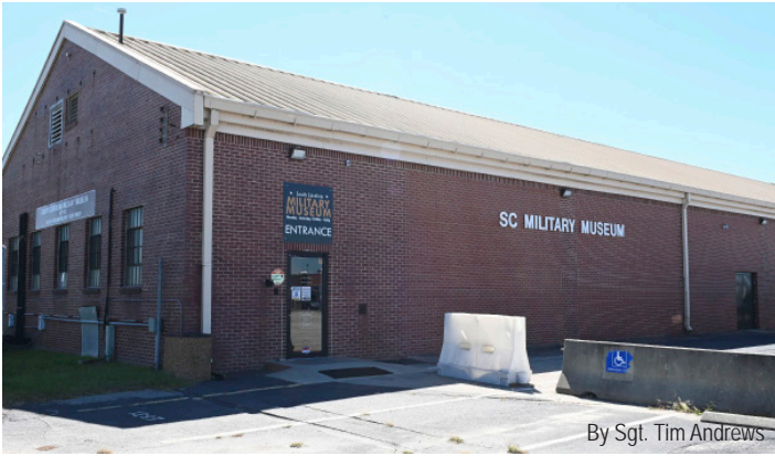
The South Carolina Military Museum is located at I National Guard Road in Columbia, South Carolina.
